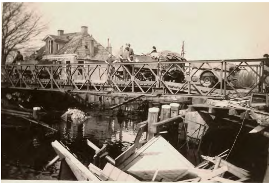
The bridge at Scharsterbrug which the three Americans had to cross, demolished by the Germans before the day before the liberation on April 16 th 1945. Canadian infantry is utilizing a temporary bailey bridge.
